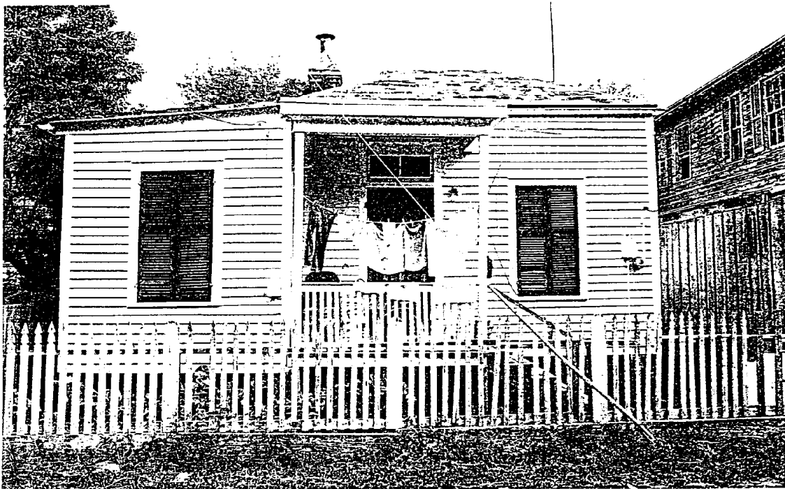
Fig. 3. 2621 Avenue K rear. Alley side of alley house with entrance oriented to the alley. Photographed circa 1977.
