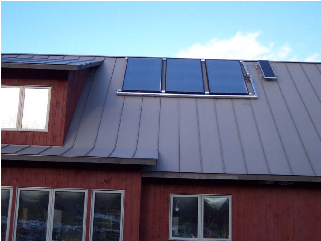
Figure 16. Flat Plate hot water collector, powered by a small Photovoltaic panel (right).
