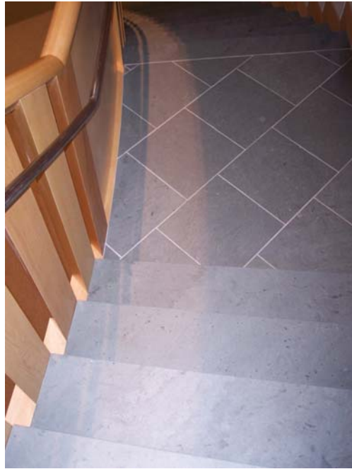
Figure 23. Local Marble, left, quarried in Danby, VT, on the exterior and local slate from Poultney, Vermont, used in the atrium and on the stairs of Middlebury College's Library.
