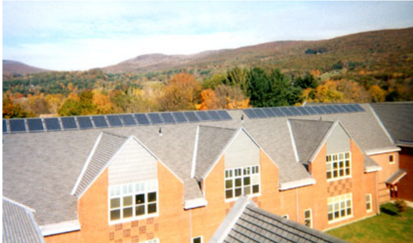
Figure 19. View of the 24 kWh Photovoltaic System on the Williamstown Elementary School. Source: http://www.williamstownelementary.org/
