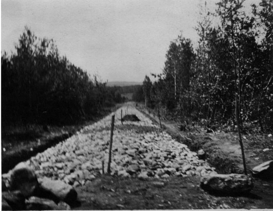
**Figure 2.8:** A section of the original Mohawk Trail highway while under construction sometime between 1912 and 1914.
