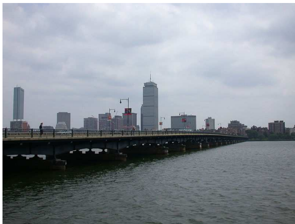
Figure: Harvard Bridge, about 620.1 meters.
