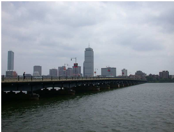
Figure: Harvard Bridge, about 620.1 meters.
