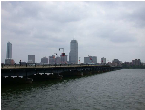
Figure: Harvard Bridge, about 620.1 meters.
