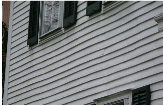
Figure 11. Siding hewn by hand.
