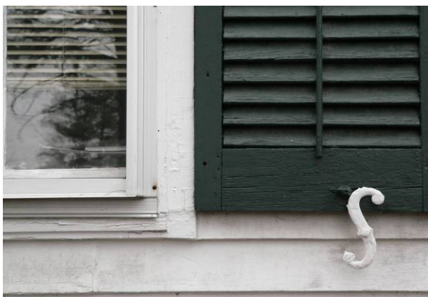
Figure 10. Original shutter hardware.
