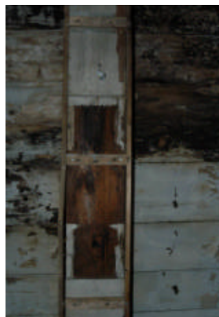
Figures 11 (left) and 12 (right): Photographs of wooden floors in building 1 showing extent of mold infestation and rot due to roof leakage. This leakage was a direct factor in the building's roof collapse in 2003.
