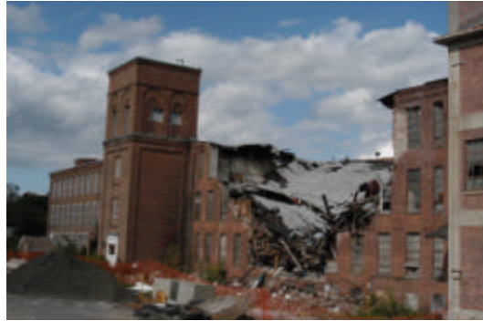
Figure 4: Photograph of Building 1 looking west showing extent of roof collapse.
